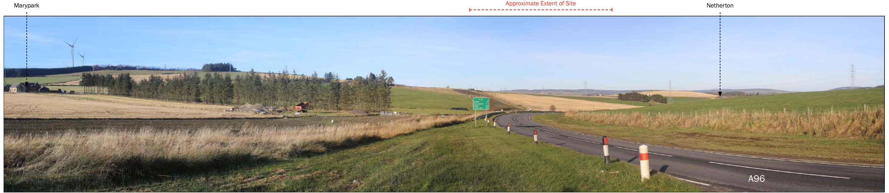
Photo Location 17: View looking north towards the site from A96/ B9115 junction
